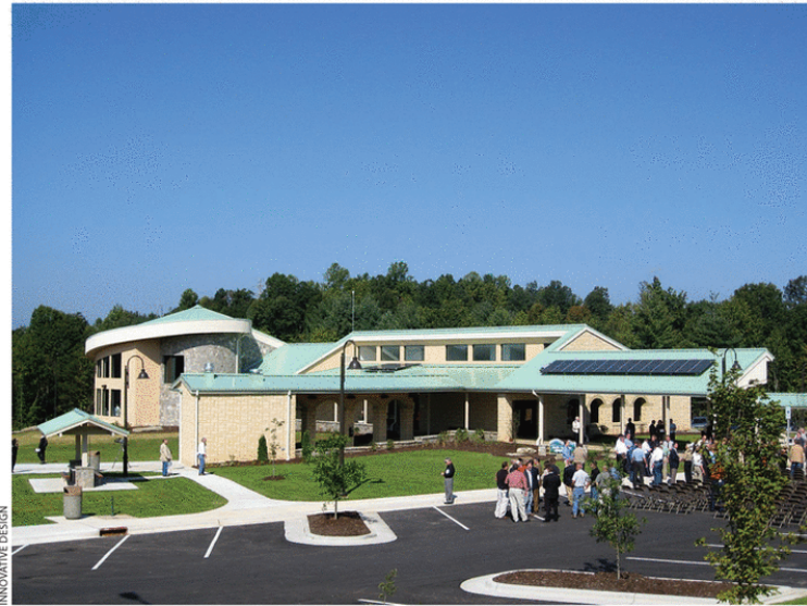
A 14-module, 3.22-kilowatt photovoltaic system is installed on the roof of the walkway canopy. Projected to generate 4,381 kWh per year, the measured annual contribution is 4,550 kWh.
